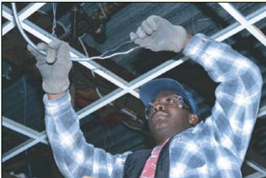
Electrical work can be deadly if not done safely.
